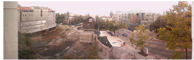
(a) Construction site of the CITRIS II building at UC Berkeley.
